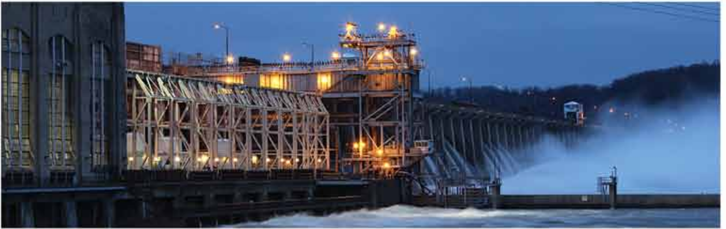
■ Hydro Power Plant
